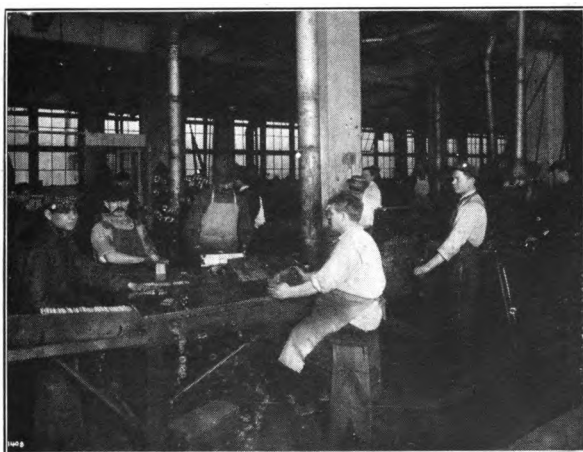
Loading the Negative Pocket with Iron Oxide.
